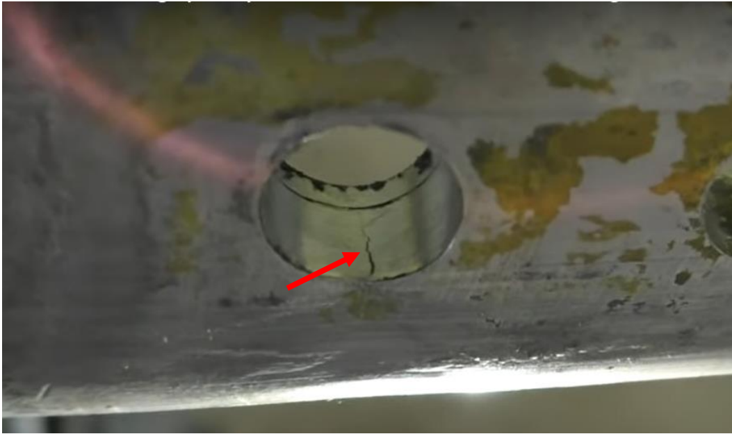
Figure 6. Example of Cracks Intersecting Bolt Hole PA-32-300, 5,319 hours TIS
